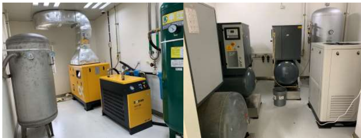
Vacuum and Compressed Air system
