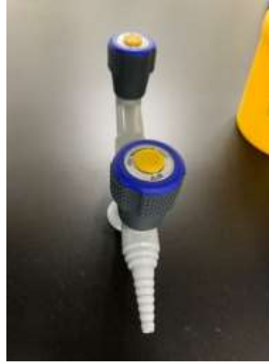
Compressed air outlet
